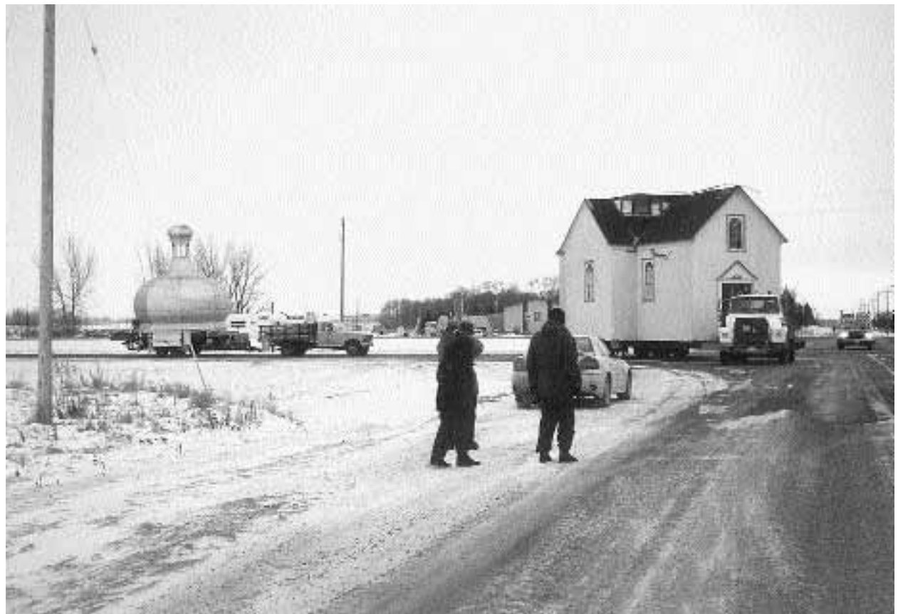
The building and dome of St. Nicholas Ukrainian Orthodox Church of Arbakka, Manitoba, are transported on flatbed trucks to Fort La Reine Museum in Portage La Prairie, some 200 miles away.
