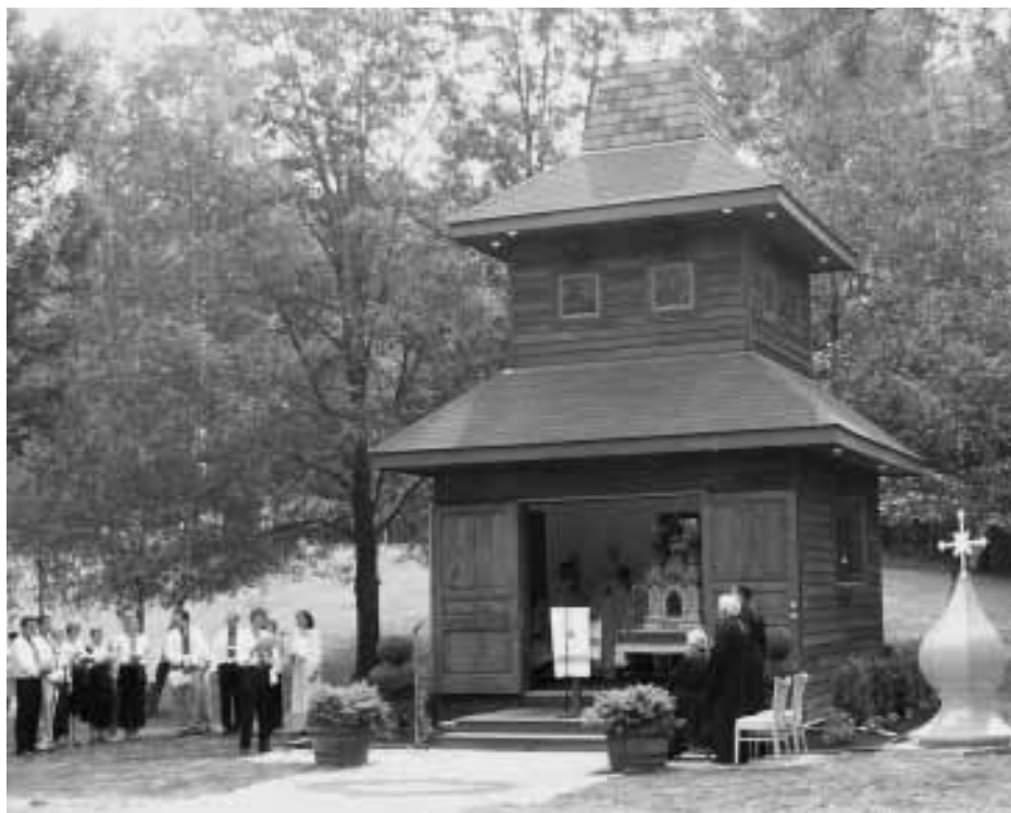
A view of the newly constructed St. Michael the Archangel Chapel.
