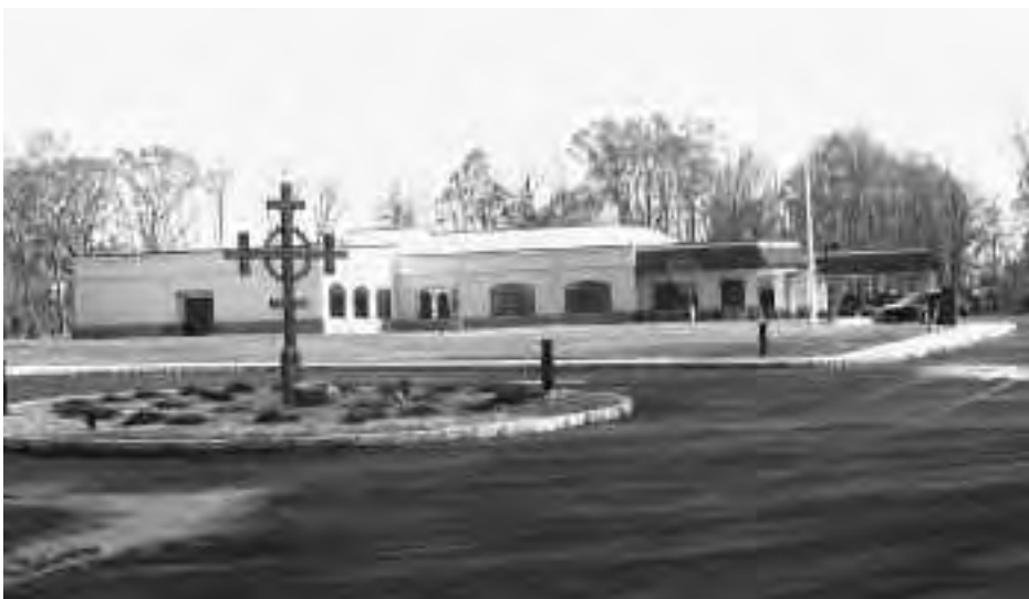
A view of the new cultural center. In the foreground is the cross erected during the groundbreaking at the site of the soon-to-be-built St. John's Church
