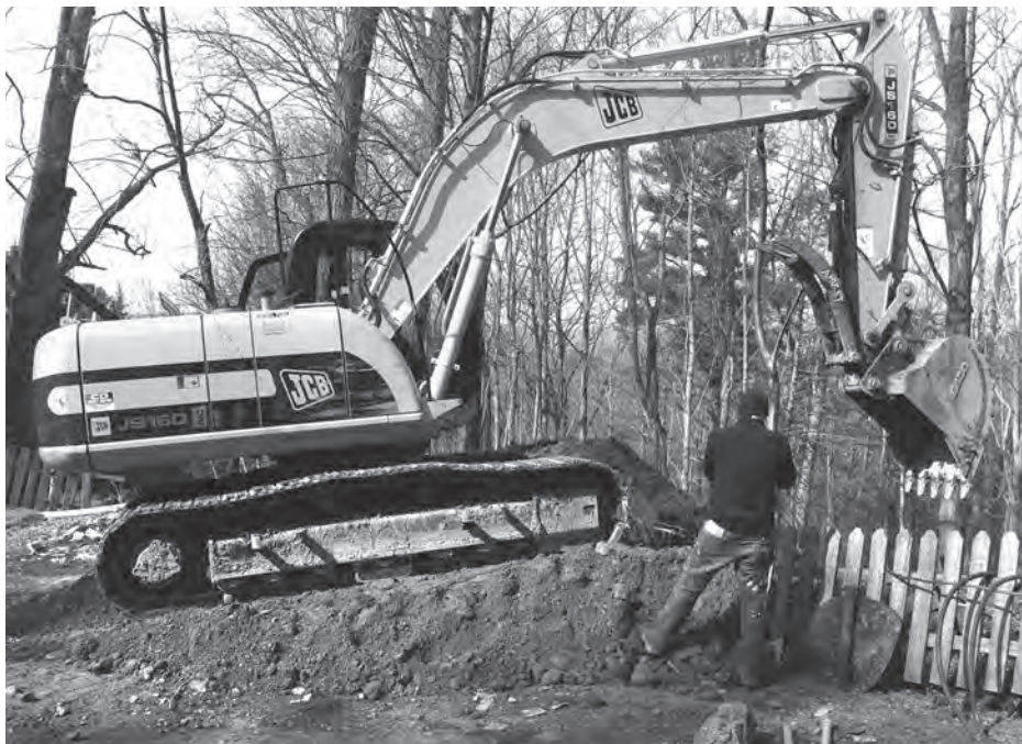
Excavation equipment on the scene at Soyuzivka.
